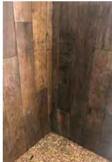
Using wood-look and pebble tile brings the outdoors in and provides a natural, earthy design to your bathroom.
